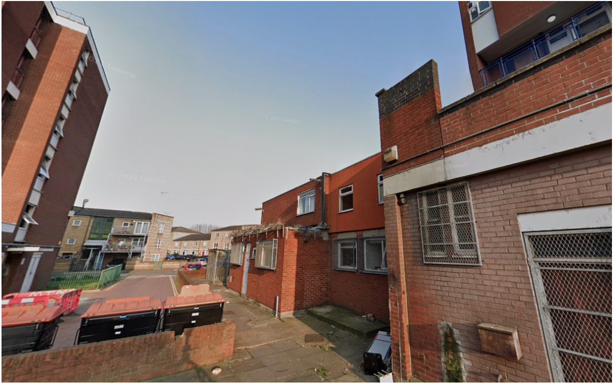
View from courtyard to rear of Kirkstead House
